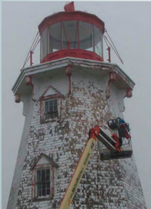
The work begins.
